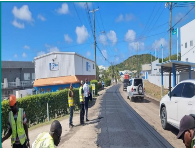
Road Rehabilitation Work - Massade Gros Islet
