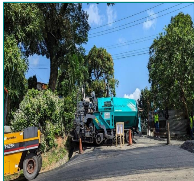
Road Rehabilitation Works - Bocage
